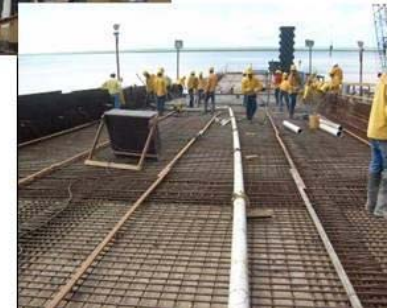
Pier access bridge
