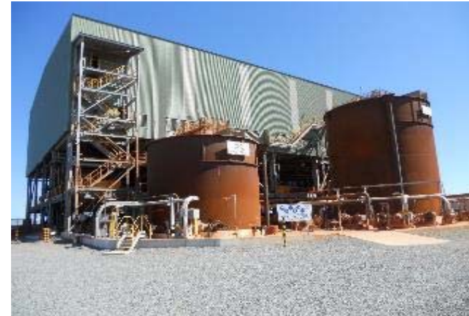
Press filtration, Western Australia
